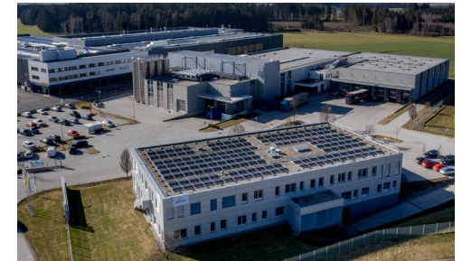
Photovoltaic system at the Rainbach site installed in 2023
