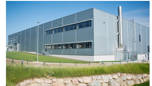
Europe's largest sterilization plant
